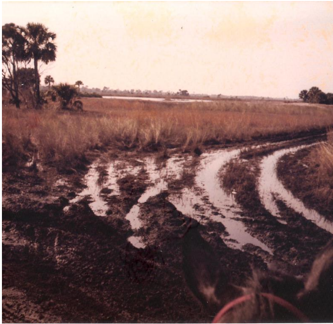
Figure 13 Swamp buggy damage in the Savannahs
